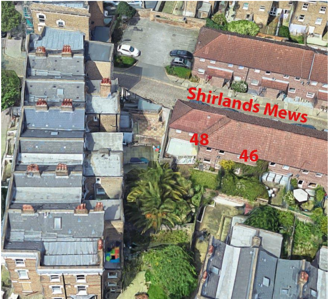
Aerial View of site
