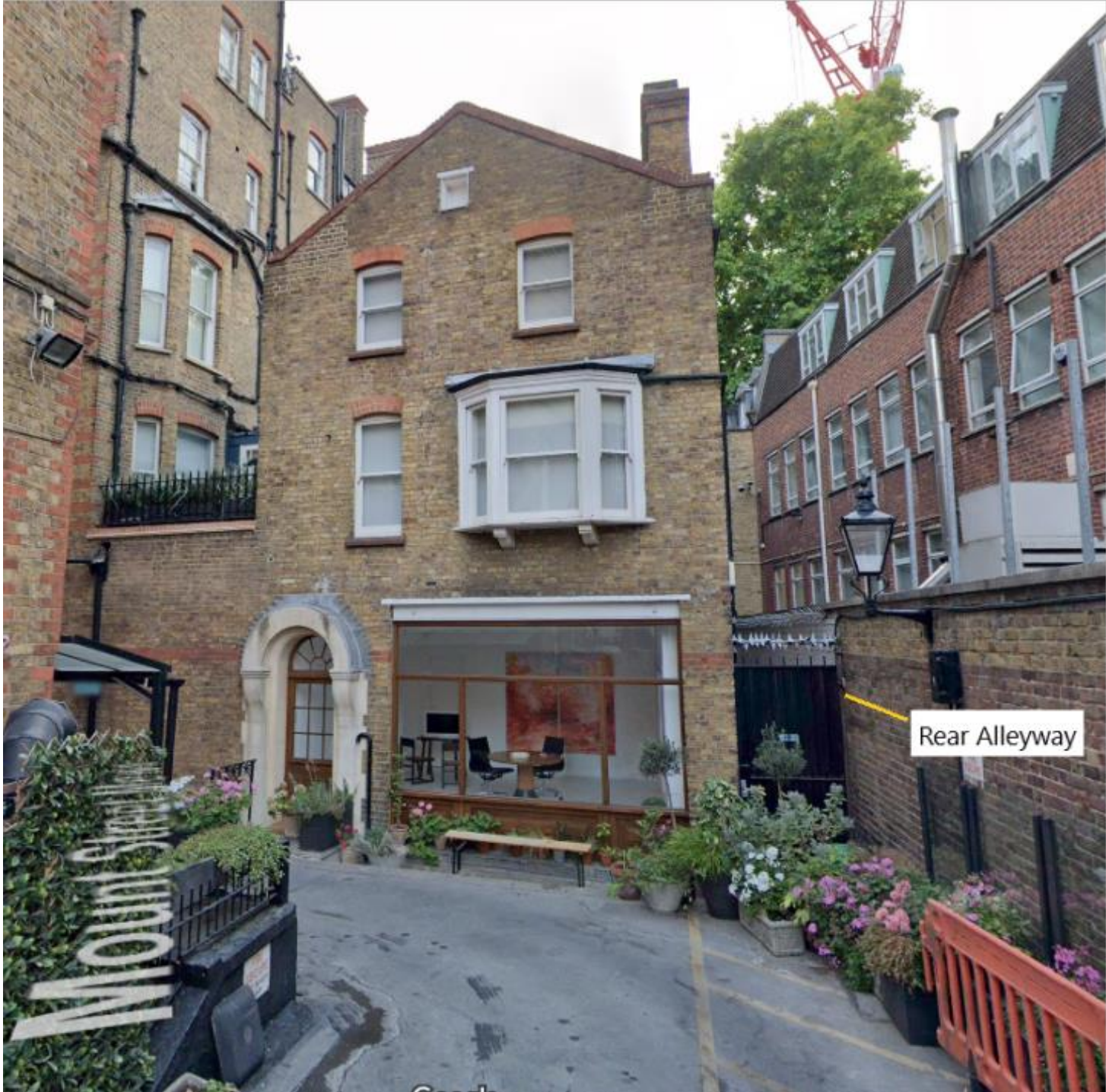
View from Mount Street Mews showing the location of the alleyway to the rear of 127 Mount Street
